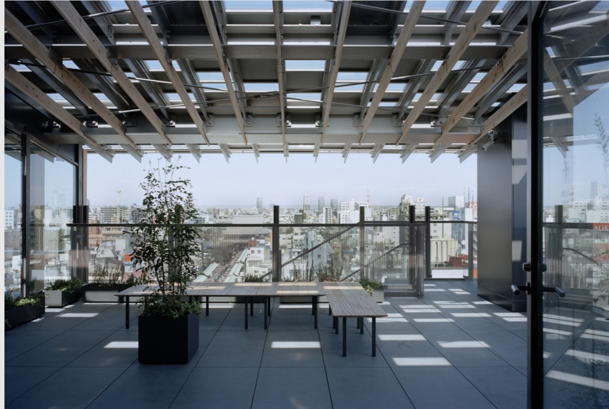
Asakusa Culture Center, Tokio, Japan / Kengo Kuma & Associates
